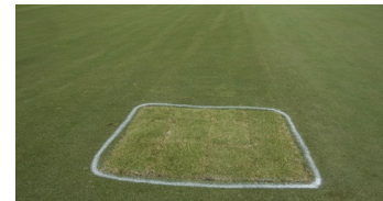
Ground under repair
